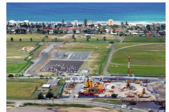
Tugun—Planned site for desalination plant
